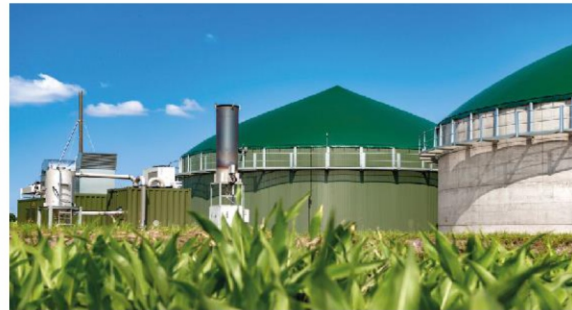
Agricultural biogas plant
